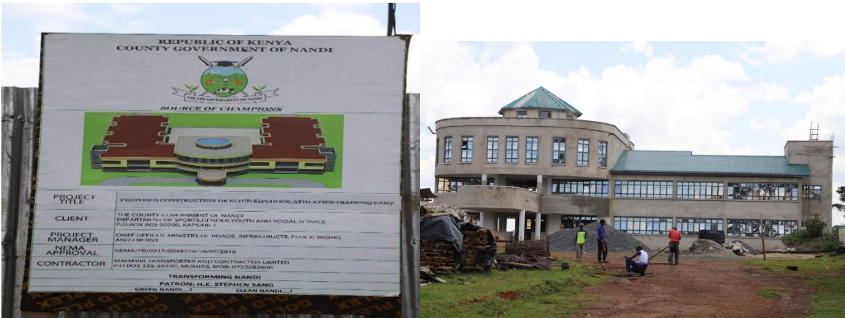
Construction of Athletic Training Camp
